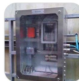
Refractometer Integrated Electronic NESTE Oil Rotterdam & Singapore
