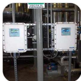
Double EEx d Refractometers BASF Group
