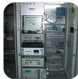
CEMS equipped with TOC & FTIR
