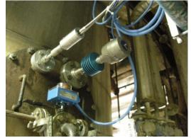
In line Viscometers
