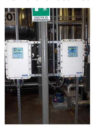
In-Line Concentration Measurement Process Refractometers
