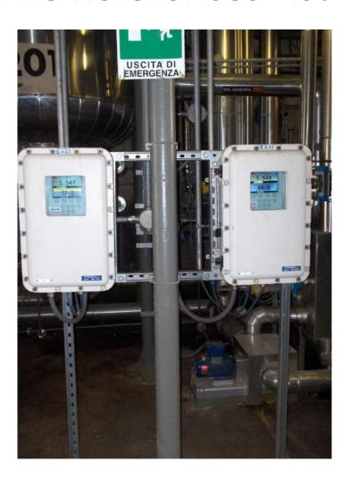
In-Line Concentration Measurement Process Refractometers
